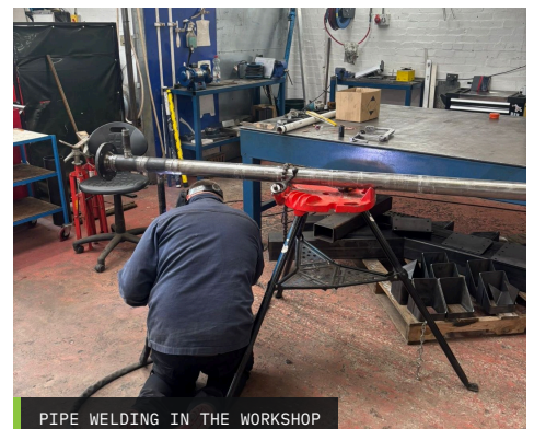
PIPE WELDING IN THE WORKSHOP
