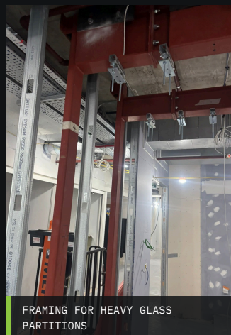
STEEL INSTALLED AT HIGH LEVEL
