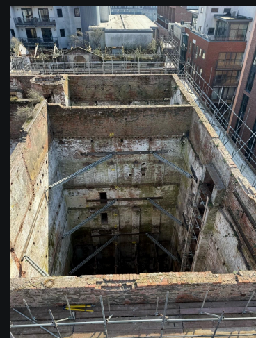
NEW STEEL WITHIN A HISTORIC SHELL
